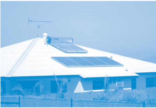
Roof-top solar PV and solar hot water heater in Palmerston.
